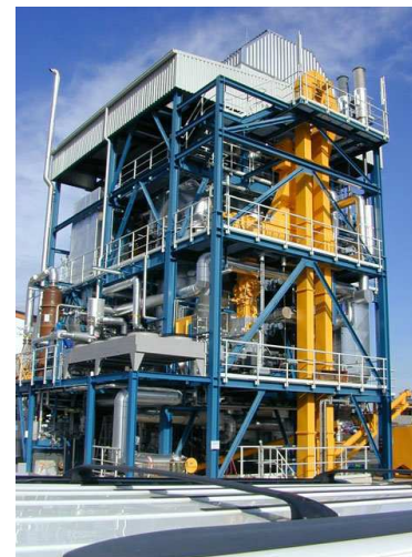
Gussing (Austria) biomass gasification plant
