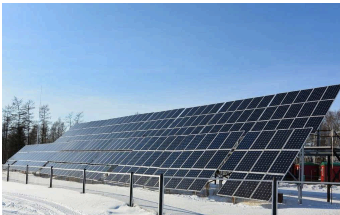
Figure 6. Batamai village solar PV system [47]
