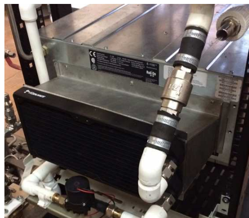
Figure 43. The view of the radiator that utilizes waste heat of the FC in H2Smart
