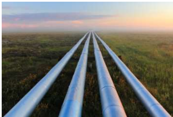
Figure 7.7 (Photo) Large diameter in-field pipelines in one technological corridor
